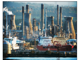
Refinery Petrochemical Plant
